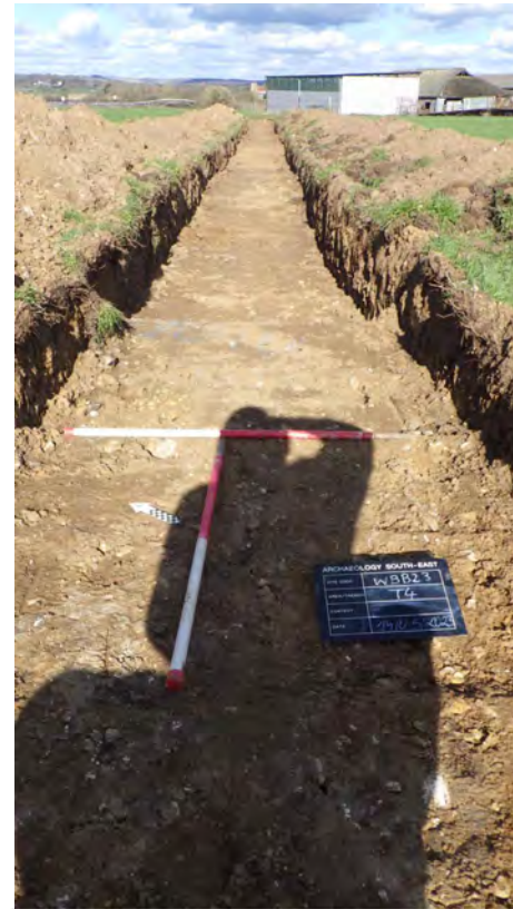
Trench 4 facing north-east
